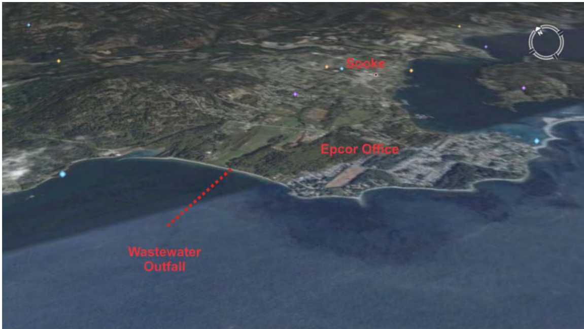
Figure 2: Aerial view of Sooke Bay outlining location of wastewater outfall with reference to Sooke and the Epcor Office.
