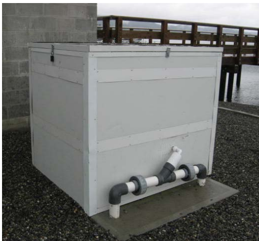
Boat Launch Odor Control for Vacuum System
