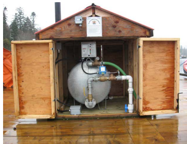
Boat Launch Sewage Vacuum Pump
