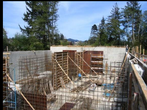
CONSTRUCTION OF INTERIOR TREATMENT PLANT WALLS
