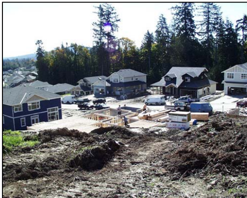
Construction in Sooke 2004
