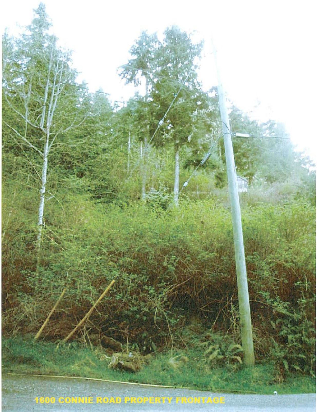
Figure 1 – Slope Assessment conducted on road right-of-way fronting 1600 Connie Rd
