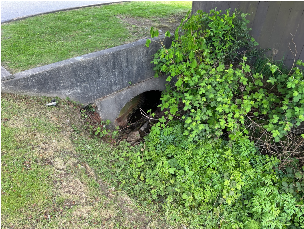
Photo 18. Upstream end of culverted section of Throup Stream, runs through Frances Gardens development (900mm to be replaced).
