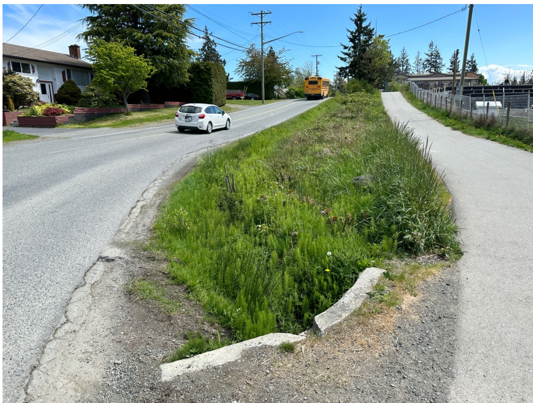
Photo 9. Ditch on west side of Church Road, to be enclosed.
