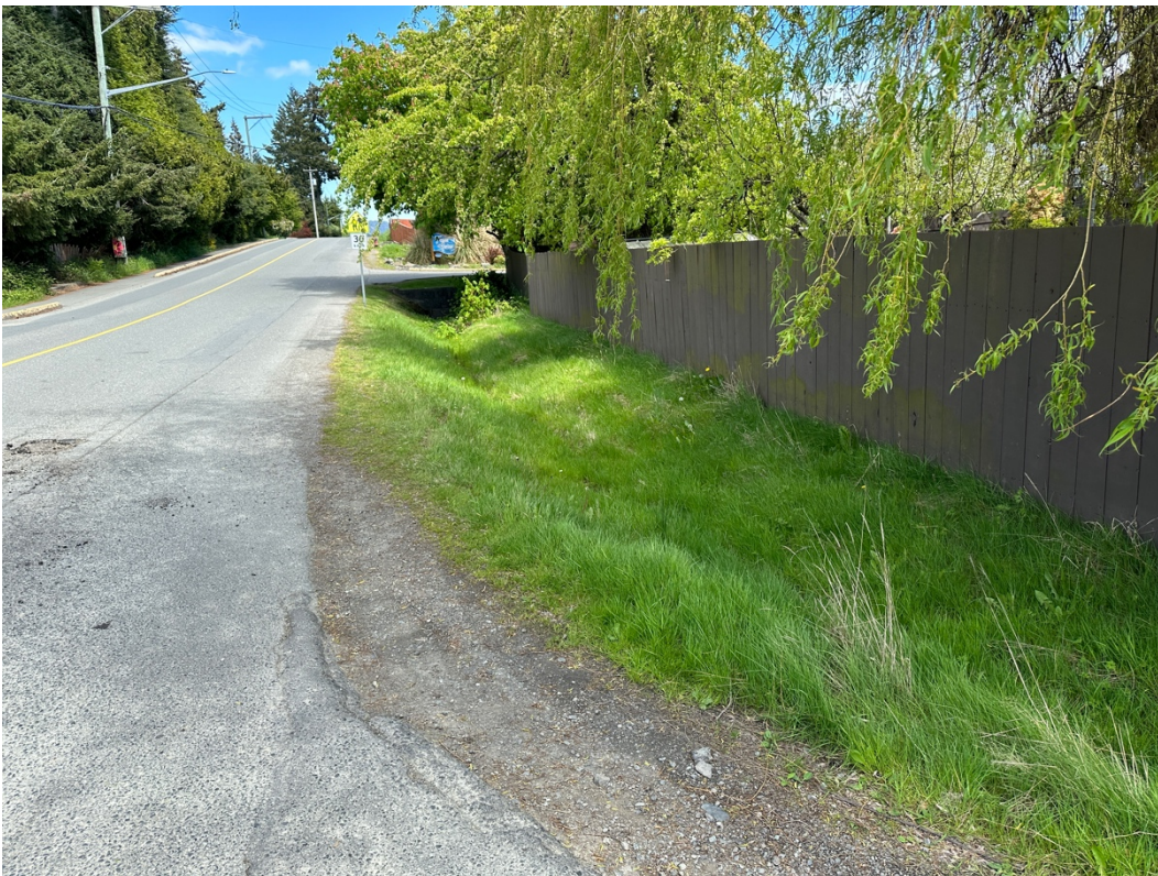
Photo 16. Short section of ditch flowing along south side of Throup Road (to be culverted), flows into Throup Stream.
