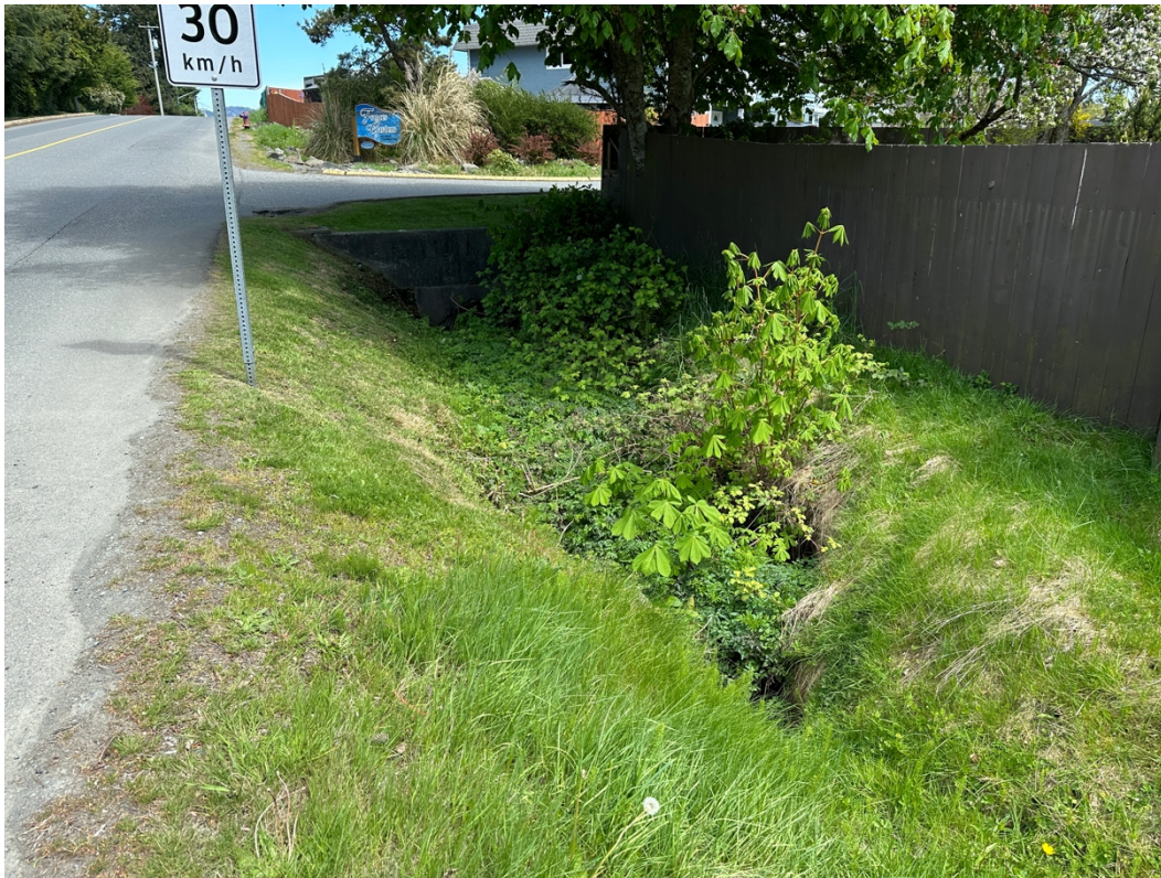
Photo 17. Short section of Throup Stream on south side of Throup Road, to be culverted and 600mm culvert under Throup Road to be replaced.
