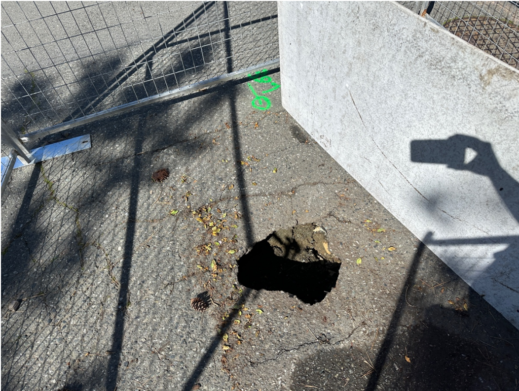
Photo 21. 900mm culvert under Throup Road, in Frances Garden, location of sink hole and required repair to the culvert.
