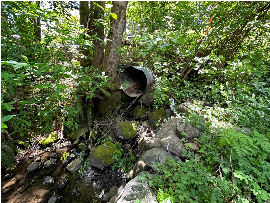
Photo 27. Downstream end of 900mm culvert under Banford Park, to be replaced, currently perched and barrier to fish passage.
