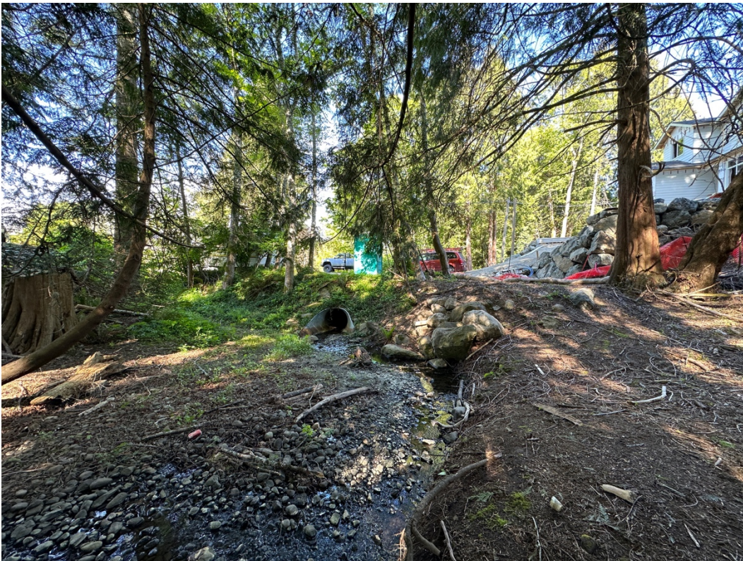
Photo 26. Throup Stream in Banford Park and upstream end of 900mm culvert under Banford Park, to be replaced.
