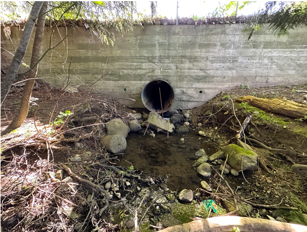
Photo 23. Downstream end 900mm culvert under Throup Road, containing Throup Stream, in Frances Garden, to be replaced, flowing into Throup Stream in Banford Park.
