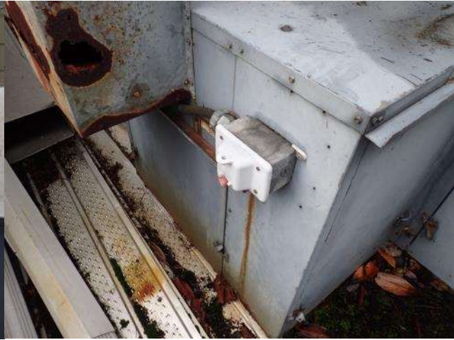
Figure 16: Municipal Hall – Abandoned makeup air unit.
