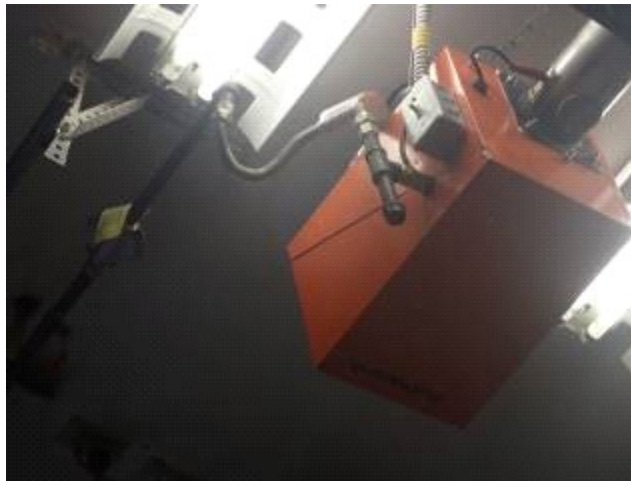
Figure 10: Fire Hall apparatus floor – radiant tube heater.
