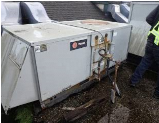
Figure 2: Packaged air-conditioner serving Fire Hall Lounge.
