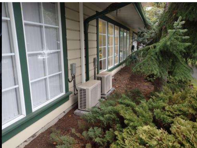
Figure 26: Municipal Hall - New condensing units.
