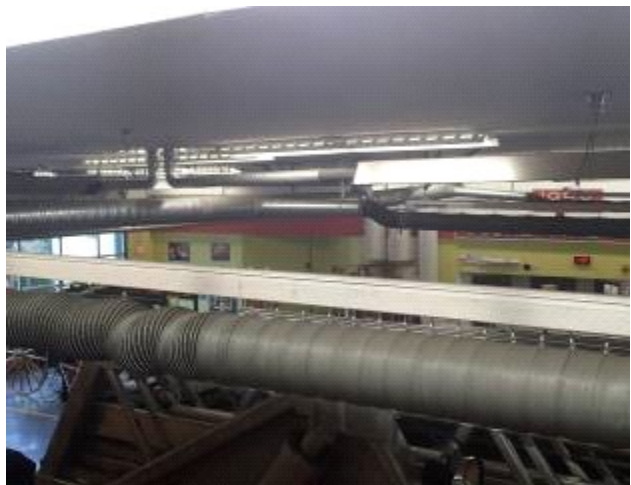
Figure 6: Fire Hall apparatus floor – vehicle exhaust ducting.
