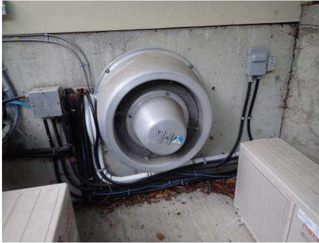
Figure 19: Municipal Hall – Washroom exhaust fan.
