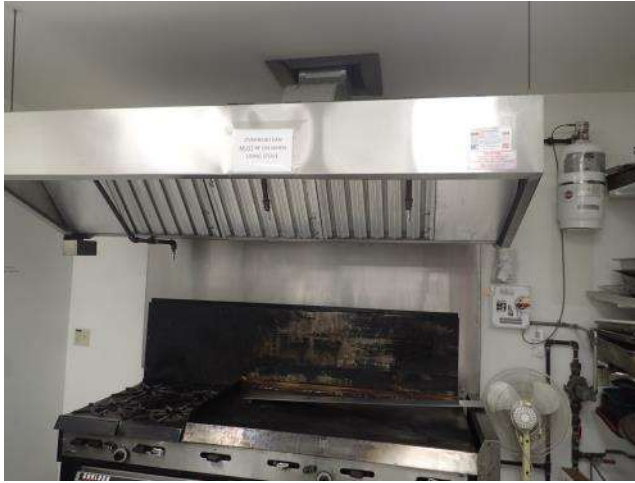
Figure 12: Fire Hall - Lounge kitchen exhaust hood.
