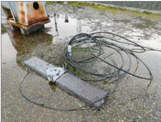
Signs of ponding, moss growth, debris, and loose wiring were noted on the BUR atop Site Building A.
