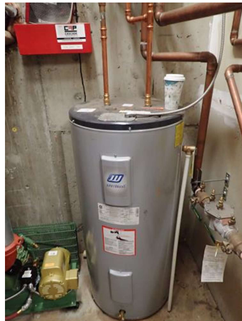
Figure 28: Municipal Hall – Domestic hot water tank.
