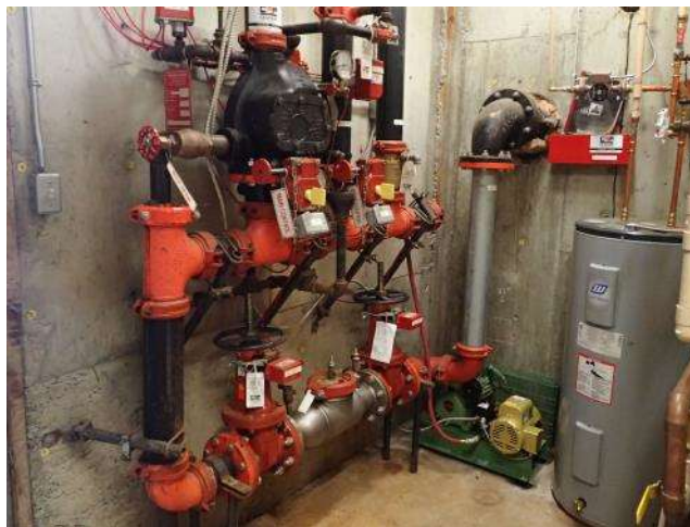
Figure 31: Sprinkler system (left), including galvanized inlet pipe and lack of fire-stopping at wall.
