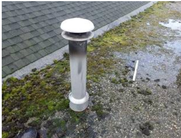
Figure 11: Fire Hall apparatus floor – radiant heater roof vent.
