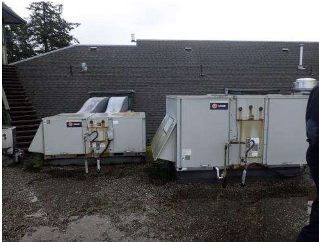
Figure 4: Packaged air-conditioners serving Fire Hall Lounge (left) and Fire Hall (right).
