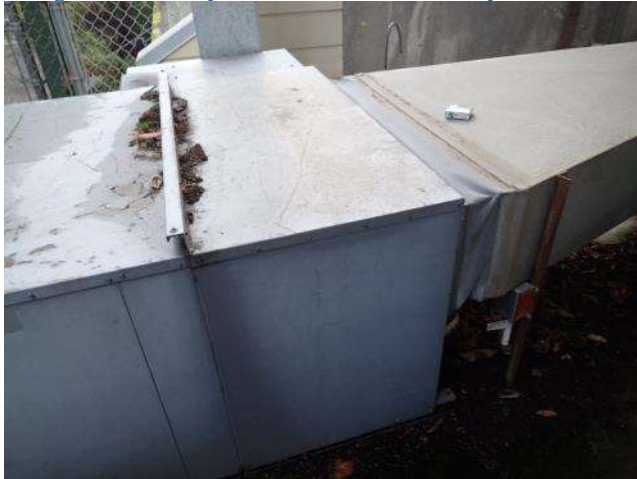
Figure 17: Municipal Hall – Abandoned makeup air unit.
