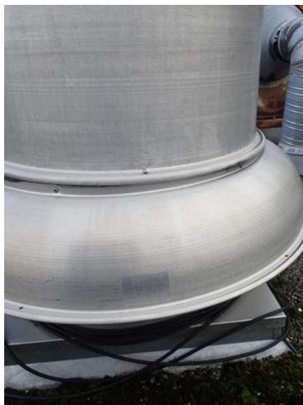
Figure 14: Fire Hall - Washroom exhaust fan.
