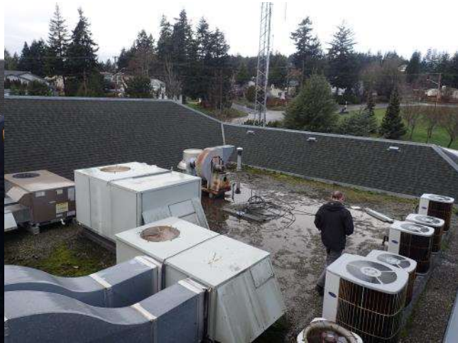
Figure 5: Packaged air-conditioners serving Fire Hall Lounge (left) and Fire Hall (right).
