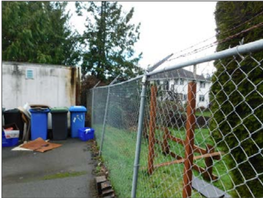
Signs of leaning were noted at localized sections of the chain-link fencing.
