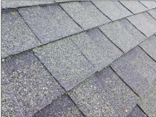
Granule loss was noted at various location of the asphalt-shingled roof system atop Site Building A.
