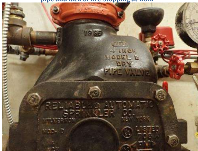
Figure 33: Sprinkler system dry pipe valve.
