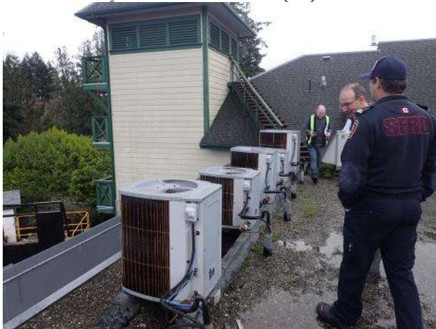
Figure 23: Municipal Hall - Some condensing units for older split systems are on fire hall roof.
