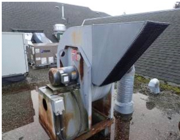
Figure 8: Fire Hall apparatus floor - exhaust fan.
