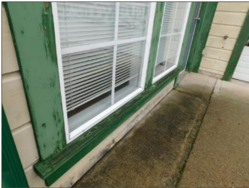
Peeling paint and localized damages were noted on the localized wooden trim boards of Site Building A.
