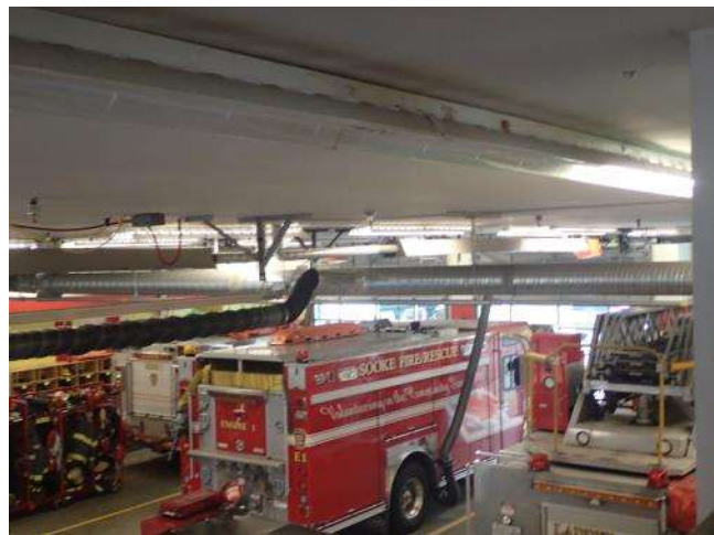
Figure 7: Fire Hall apparatus floor – vehicle exhaust ducting.
