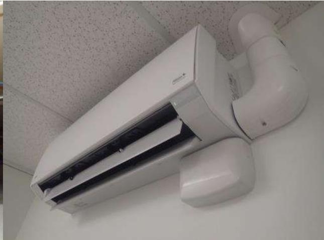
Figure 22: Municipal Hall - Typical wall-mounted split system, indoor unit (new).
