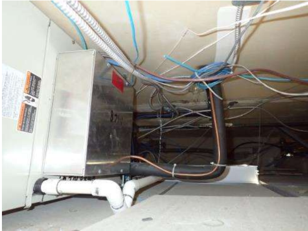
Figure 21: Municipal Hall - Typical ceiling-mounted split system ducted indoor unit (old).
