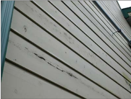
Peeling paint and localized damages were noted on the wood siding of Site Building A.
