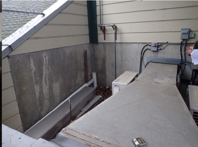
Figure 18: Municipal Hall – Makeup air duct.
