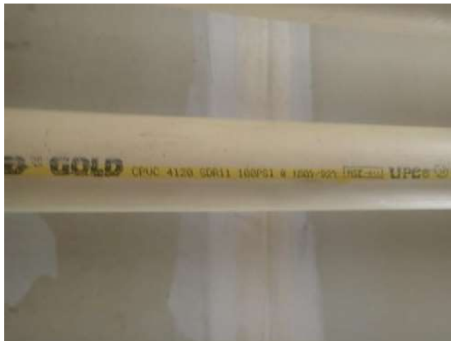
Figure 29: cPVC piping, typical of domestic water distribution piping throughout building.
