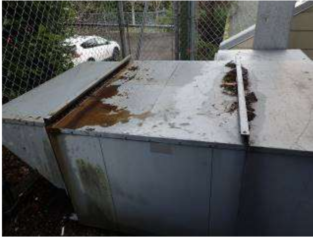
Figure 15: Municipal Hall – Abandoned makeup air unit.
