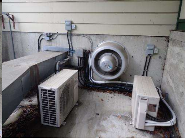
Figure 20: Municipal Hall – Washroom exhaust fan, adjacent to makeup air duct. Possibly suitable to replace both with a heat recovery ventilator.
