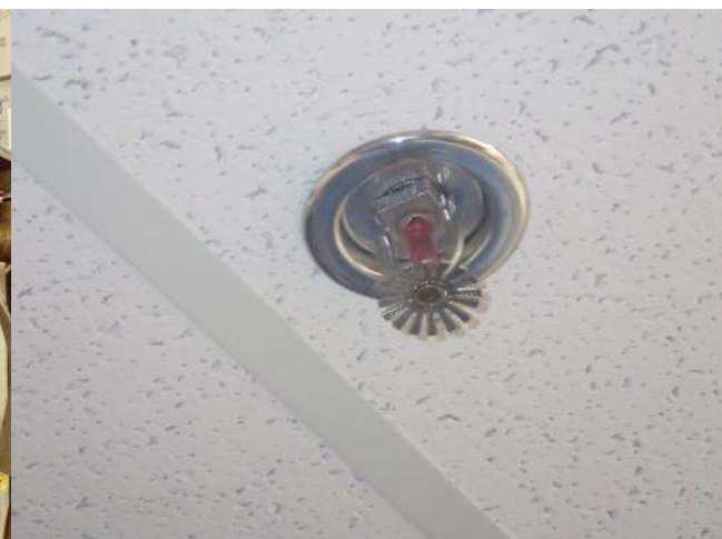
Figure 34: Typical sprinkler head in office space. Coverage not compliant with code in some areas.
