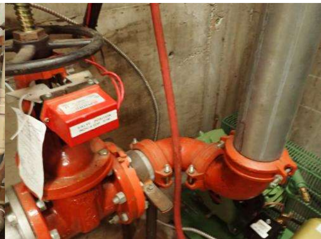
Figure 32: Sprinkler system - valve with recent test tag.
