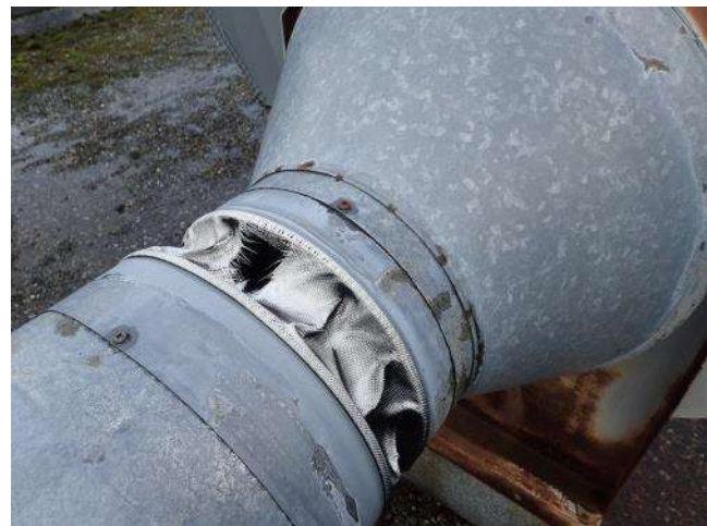
Figure 9: Fire Hall apparatus floor - exhaust fan/flexible connector.
