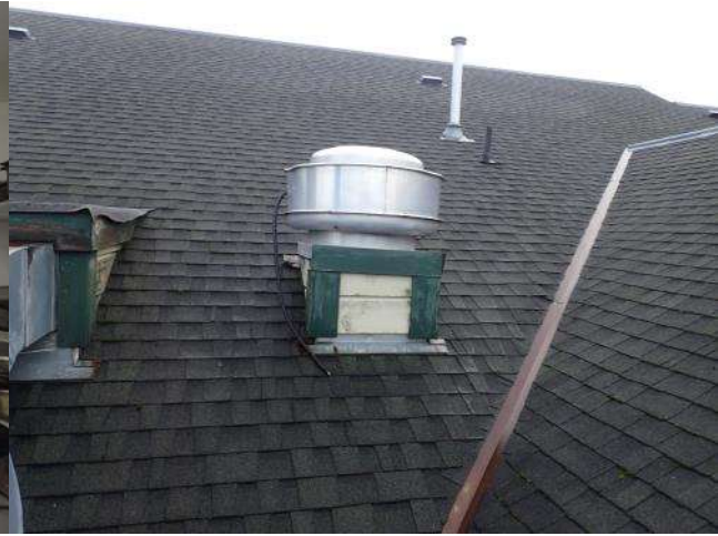
Figure 13: Fire Hall - Lounge kitchen exhaust fan.
