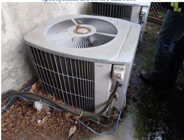
Figure 25: Municipal Hall - Additional condensing units, located adjacent to makeup air unit.
