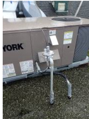
Figure 3: New packaged air-conditioner serving council chambers.
