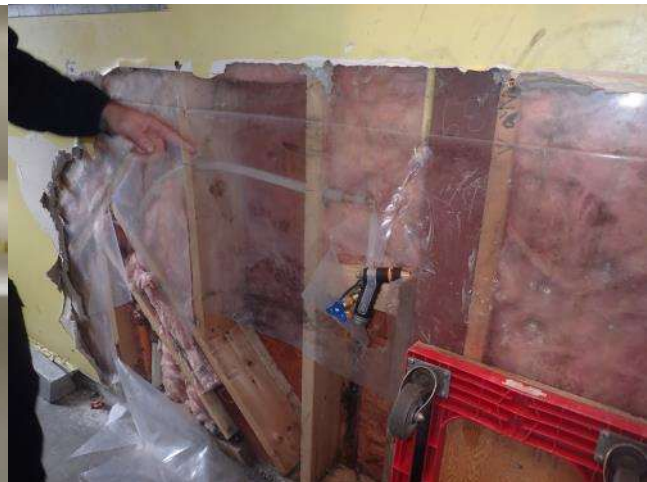
Figure 30: Fire Hall - Hose bib piping replacement due to failed cPVC domestic cold water piping.
