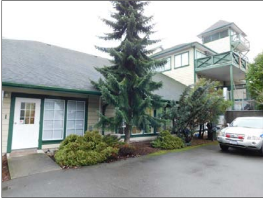
Partial view of the north elevation of Site Building A.
