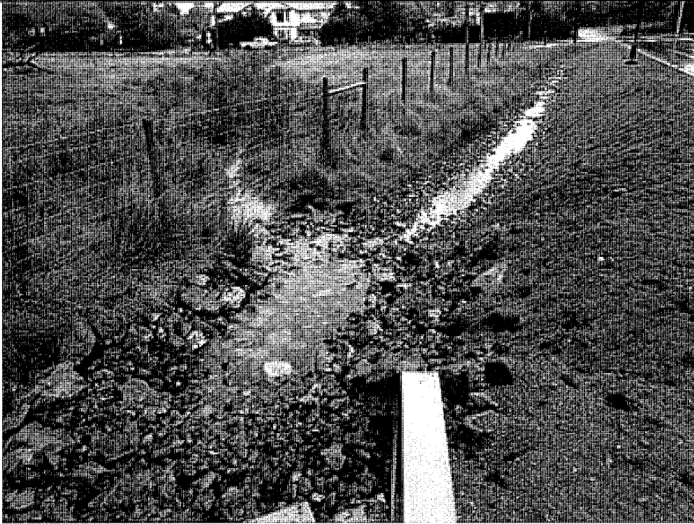
SE ditch drains toward top of picture across the corner of the property
