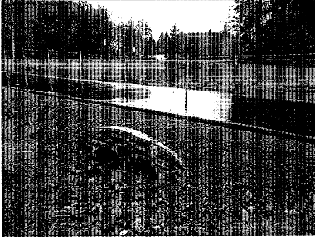
The ditch seen from the d/s end of new asphalt walkway along w side of Church Rd.
