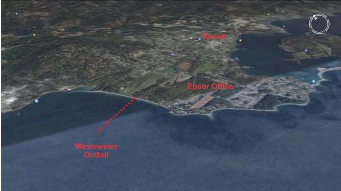
Figure 2: Aerial view of Sooke Bay outlining location of wastewater outfall with reference to Sooke and the Epcor Office.
