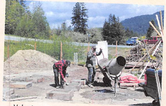
Volunteers pouring foundation for Apple Shack
