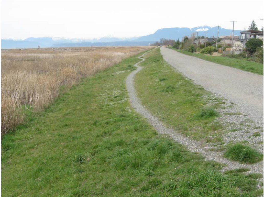
Figure 1-9: View of Seaward Face
