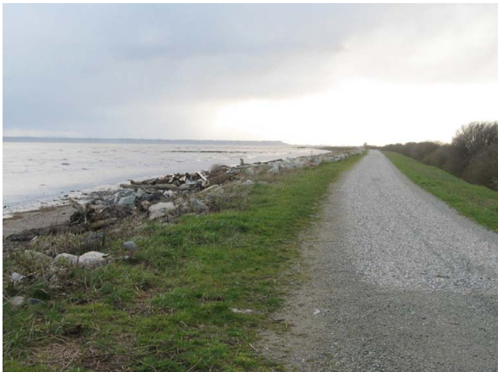
Figure 1-4: View looking W along Existing Dike Crest
