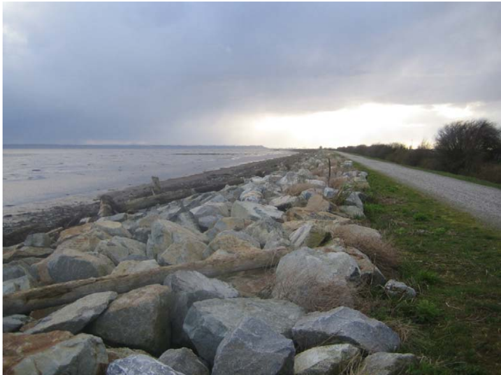
Figure 1-3: View Looking W along Seaward Face of Dike
